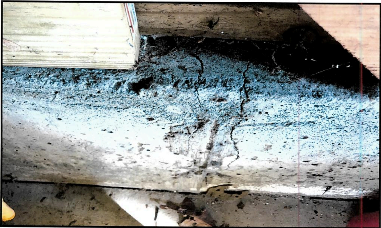
PHOTO 4: 7/13/2021 – Interior Vertical Crack in Garage Foundation Wall.
