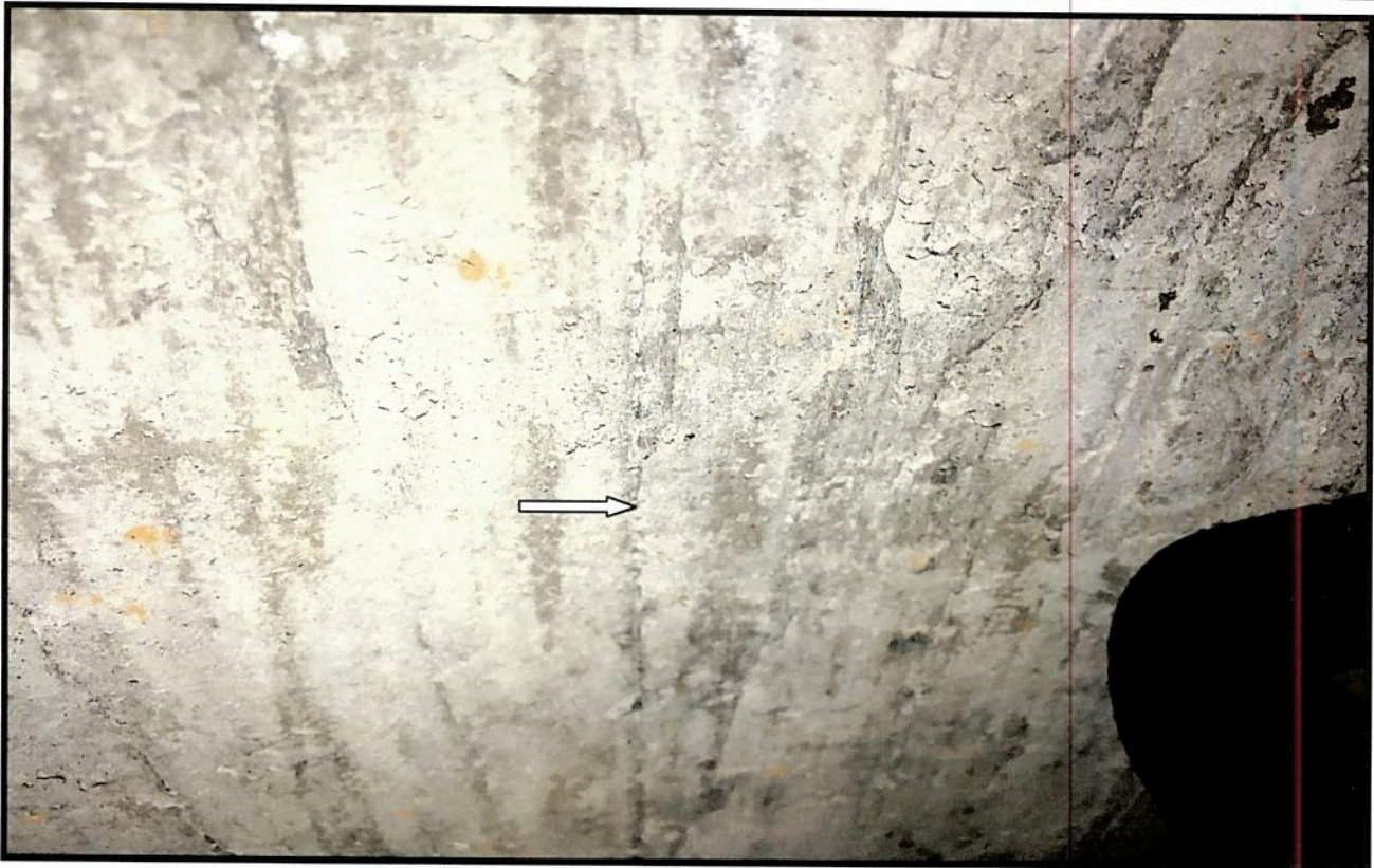
PHOTO 3: 7/13/2021 – Interior Vertical Basement Wall Crack.
