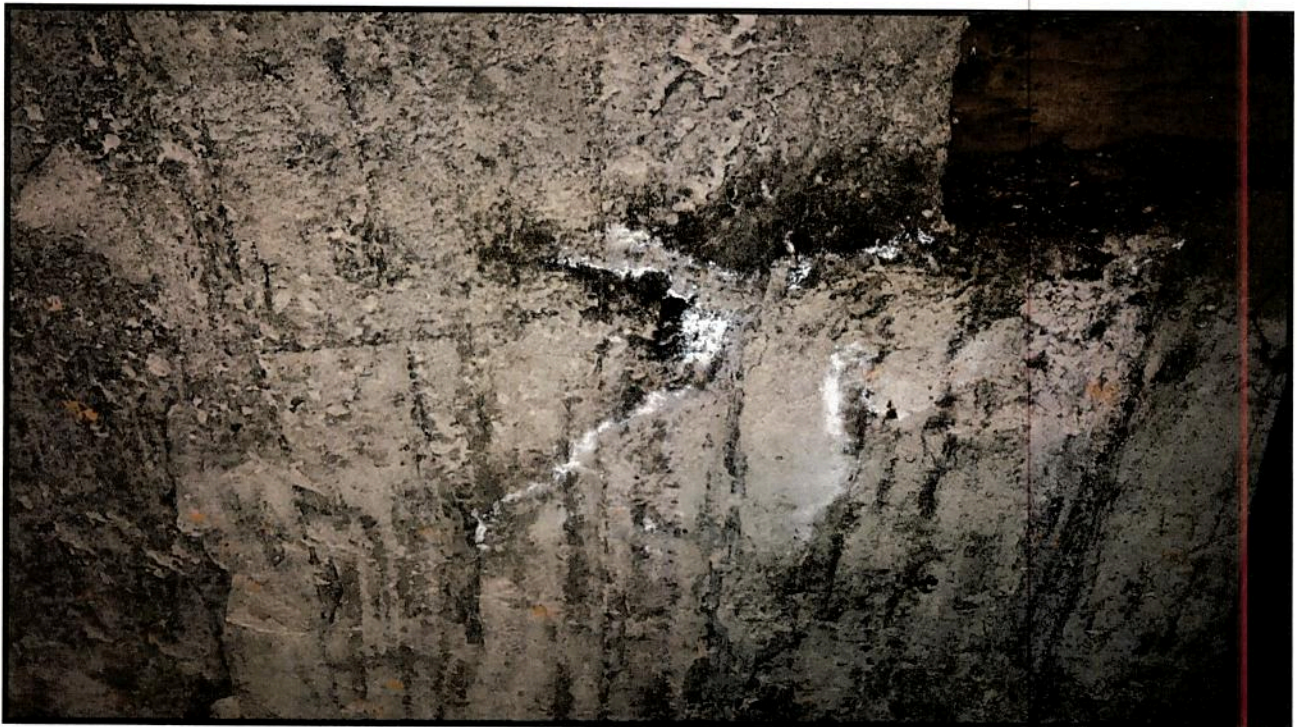
PHOTO 2: 7/13/2021 – Interior Diagonal Cracking and Efflorescence at Wall Step.
