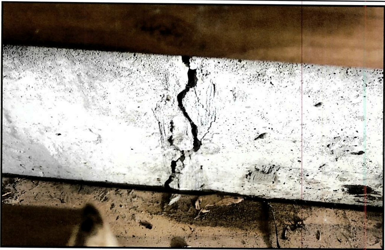
PHOTO 5: 7/13/2021 – Interior Settlement Crack in Garage Foundation Wall.
